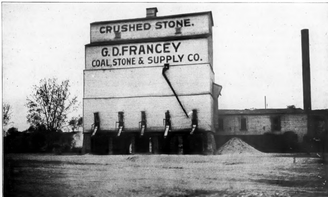
The Storage Unit of the G. D. Francey Coal, Stone and Supply Company. Note the Easy Access for Trucks
